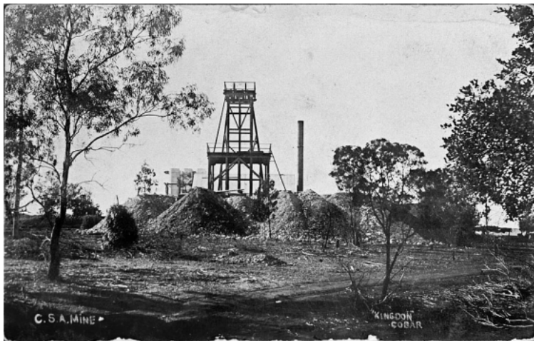
New three compartment main shaft at the C.S.A. circa 1908 from the west.
